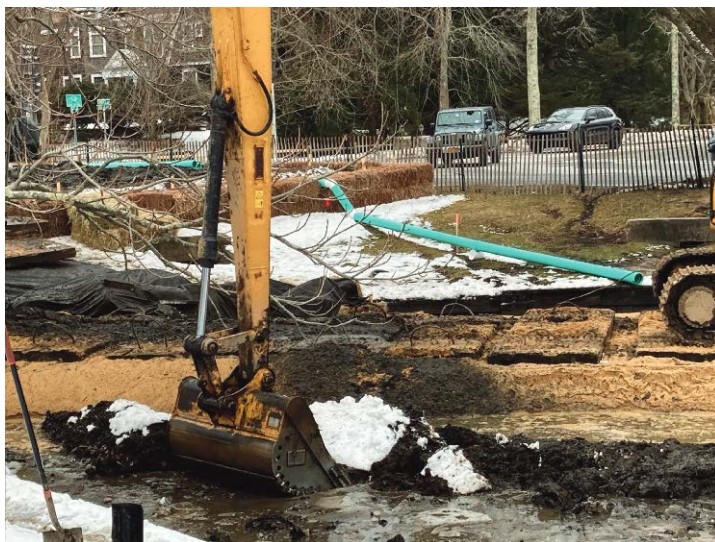
Dredging continues and should wrap up by late spring.
